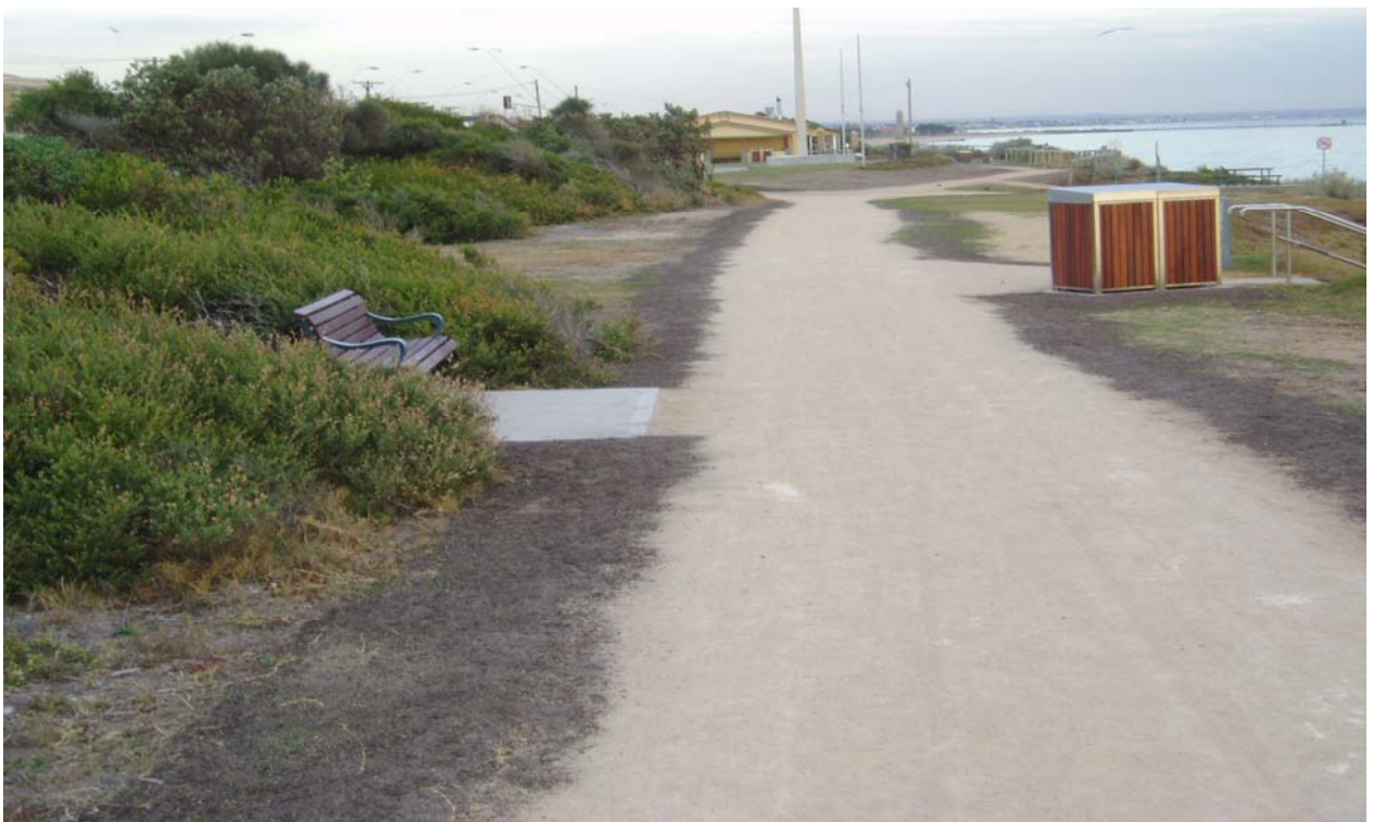
View to south-east from near Surf Street, Parkdale, showing 2.5 metre wide bicycle road
