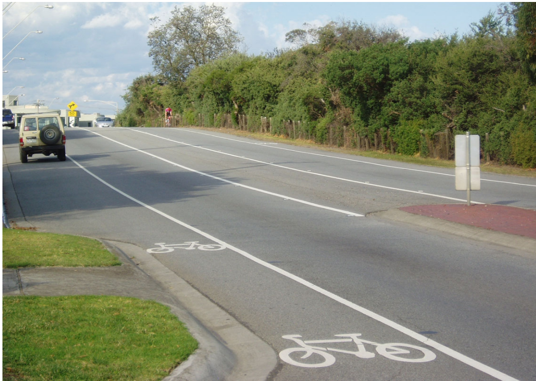
Safety Section ( Traffic Control Zone ), opposite 23 Beach Road, Beaumaris, from Wells Road to Cliff Grove, 2007-11-18
